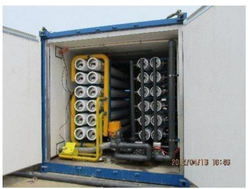
4. Close up view of RO membranes and high pressure pipe work.
